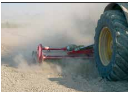
Work in difficult conditions.
